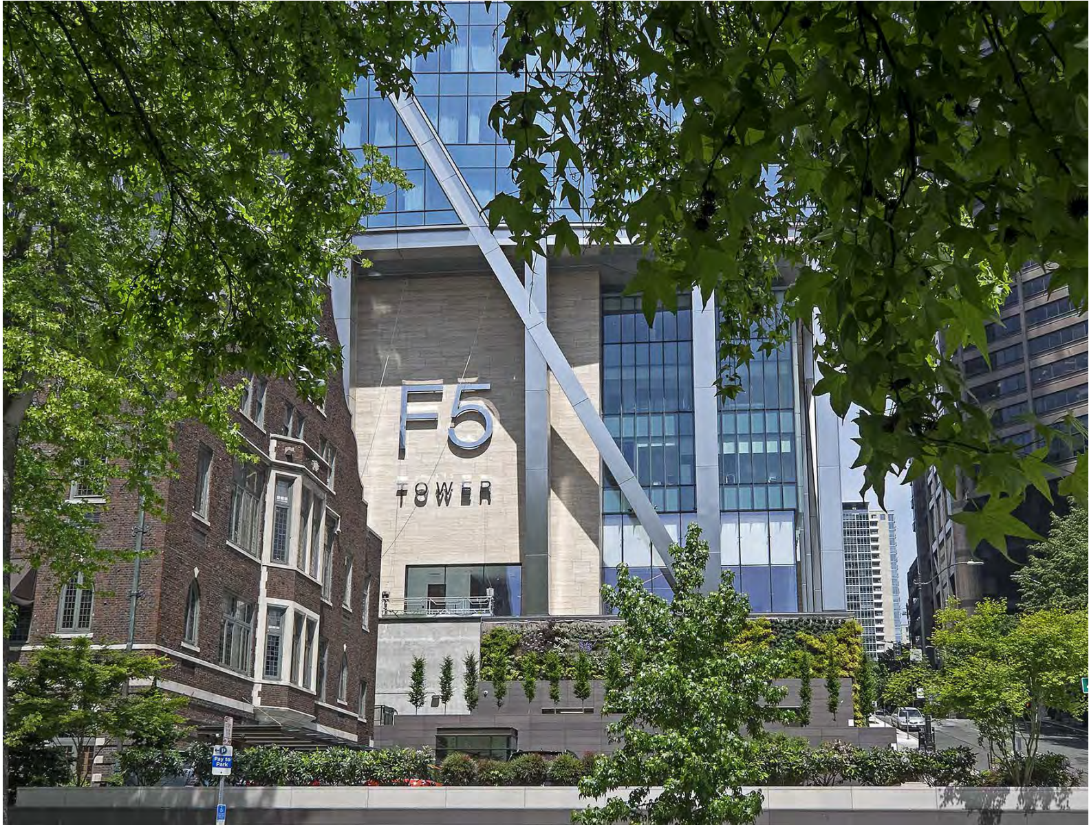
F5 TOWER - SEATTLE WA
